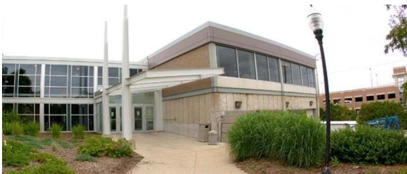
Blackhawk Commons – a University of Wisconsin student food services building. Photograph by Jeff Hill, Sr.
