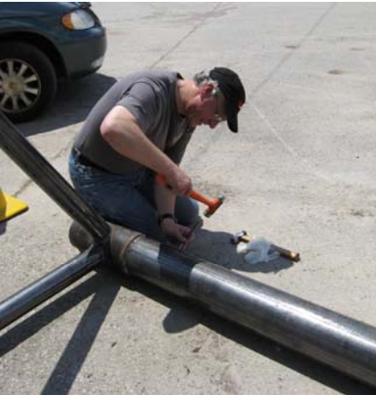
EAA 932 member Steve Mark tapping his name into a leg of the way finding tower after he finished welding on it.
